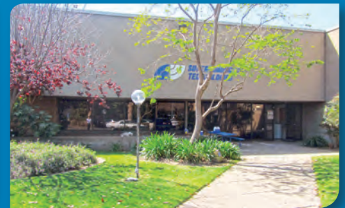
460 Ward Dr., Goleta Industrial/Warehouse | 9,500 SF Leased to Deployable Space Systems
